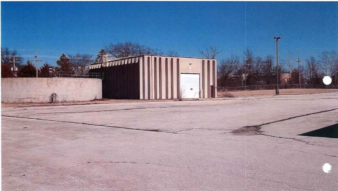
Tyson Facility – Wastewater Treatment Plant
