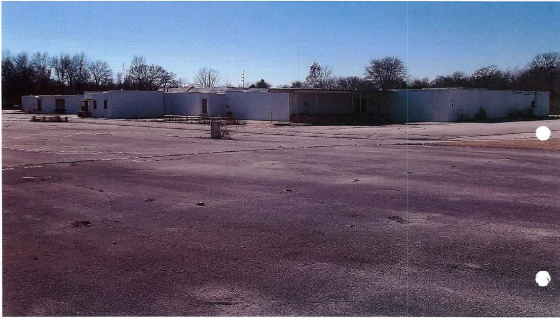
Tyson Facility – North and East Sides
