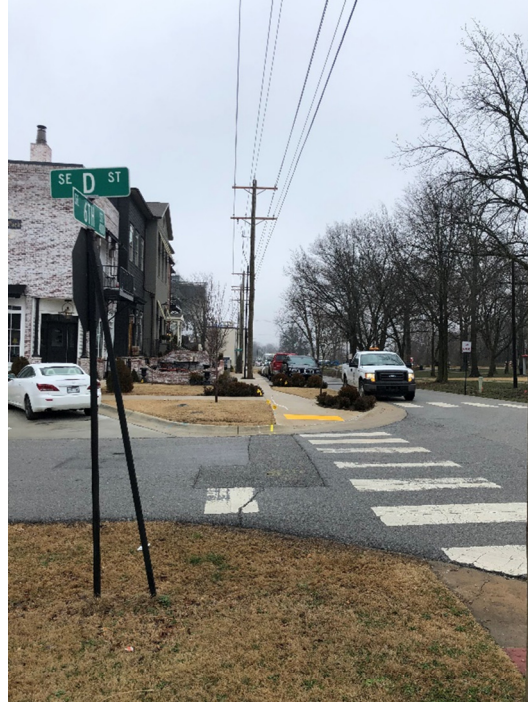
No Stop Control on SE 6 th St. Parallel parked cars are within sight triangle.
