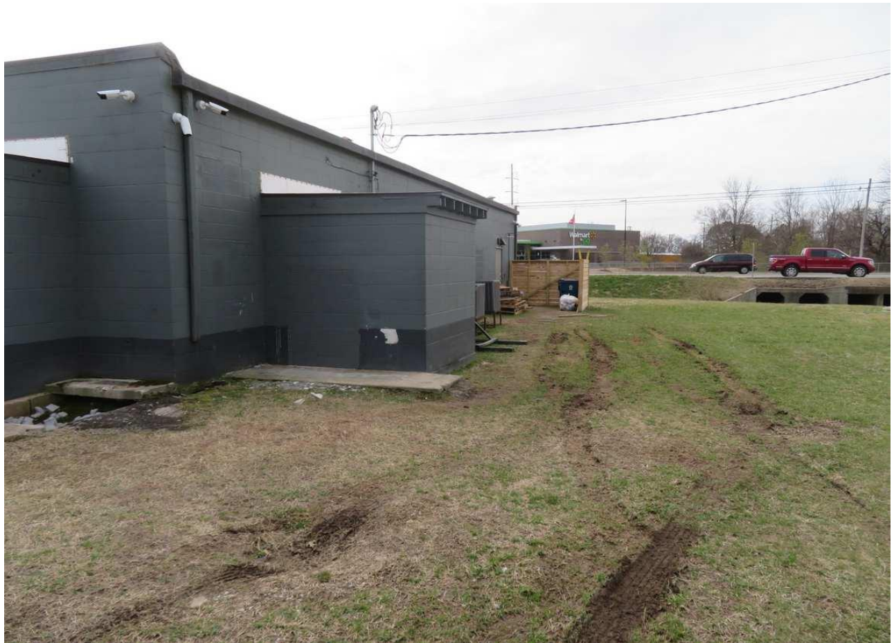
Looking westerly at the back of the building (proposed delivery driveway to the back door).
