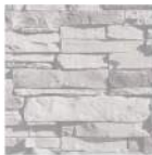
NATURAL STONE MASONRY
