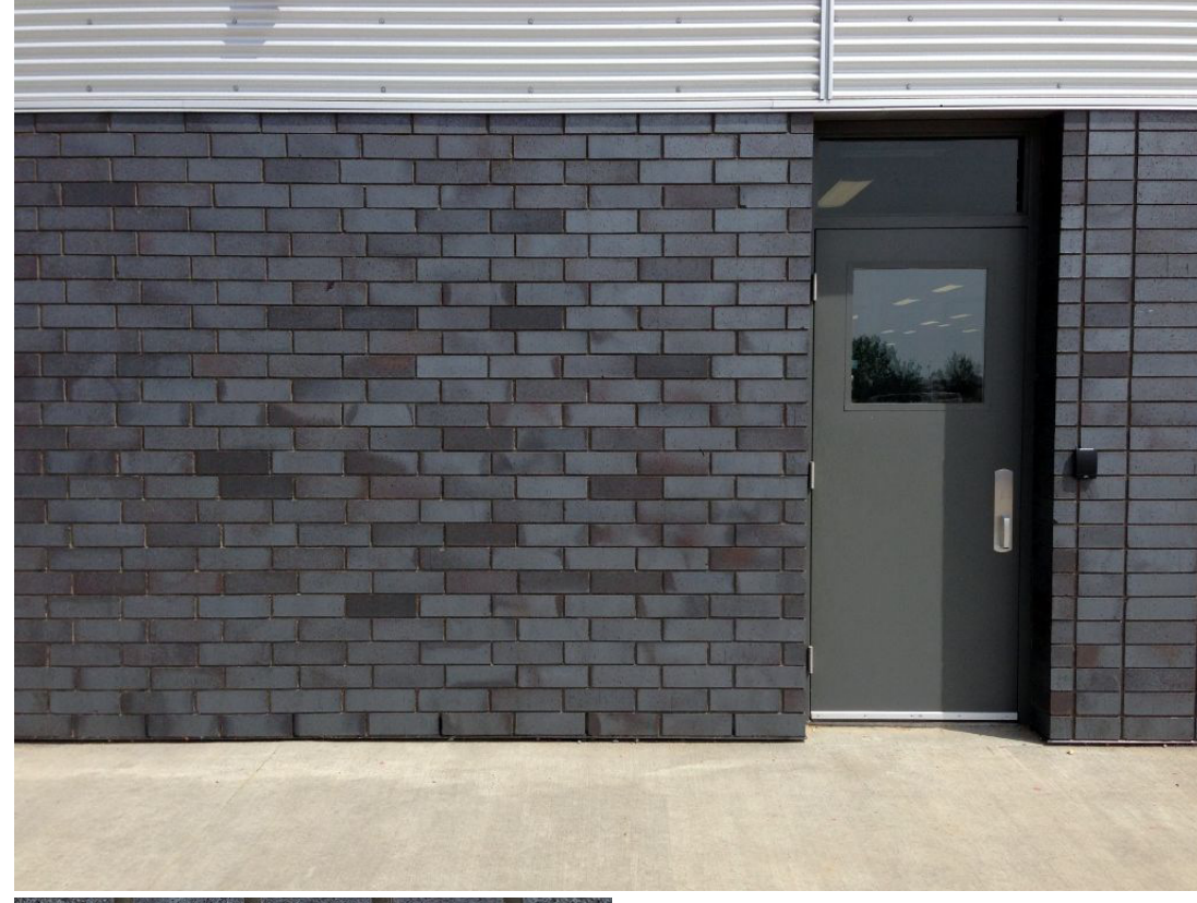
BRICK THIN-BRICK INSET INTO PRECAST PANEL COLOR: EBONITE VELOUR
