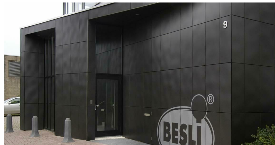
PROPOSED PRELIMINARY PRODUCT - EQUAL TO TRESPA METEON PANEL (5/16" THK. THERMOSET FIBER RESIN LAMINATED PANEL) METALLICS - M21.8.1 - GRAPHITE GREY - SATIN
