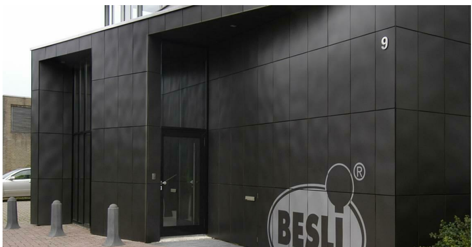
PROPOSED PRELIMINARY PRODUCT - EQUAL TO TRESPA METEON HPL (HIGH PRESSURE LAMINATE) PANEL METALLICS - M21.8.1 - GRAPHITE GREY - SATIN
