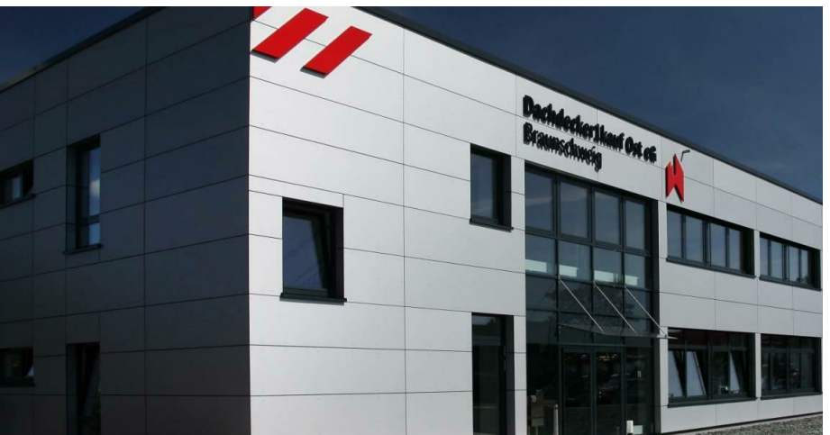
PROPOSED PRELIMINARY PRODUCT - EQUAL TO TRESPA METEON HPL (HIGH PRESSURE LAMINATE) PANEL METALLICS - M51.0.1 - ALUMINUM GREY - SATIN
