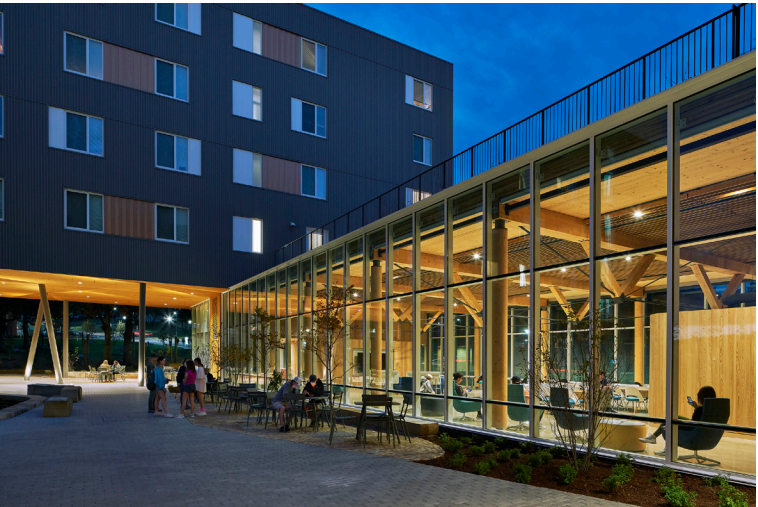
Adohi Hall in Fayetteville, expressing the quality of mass timber in community spaces and housing.
