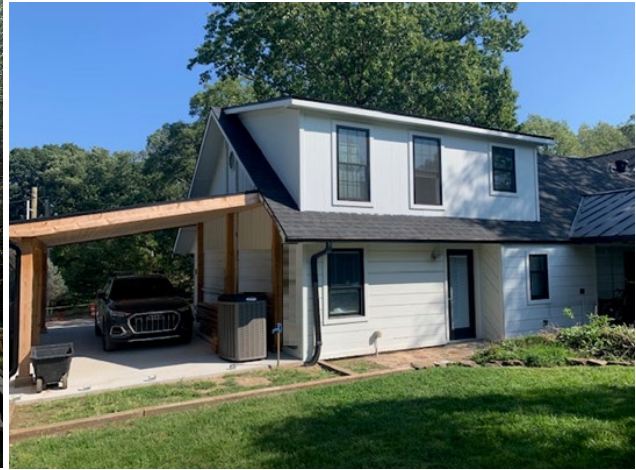
Pic2. New carport on the same existent slab
