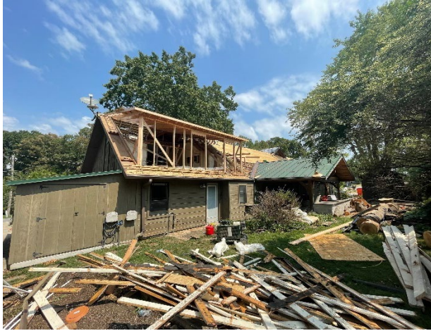
Pic1. Old shed (already demolished)
