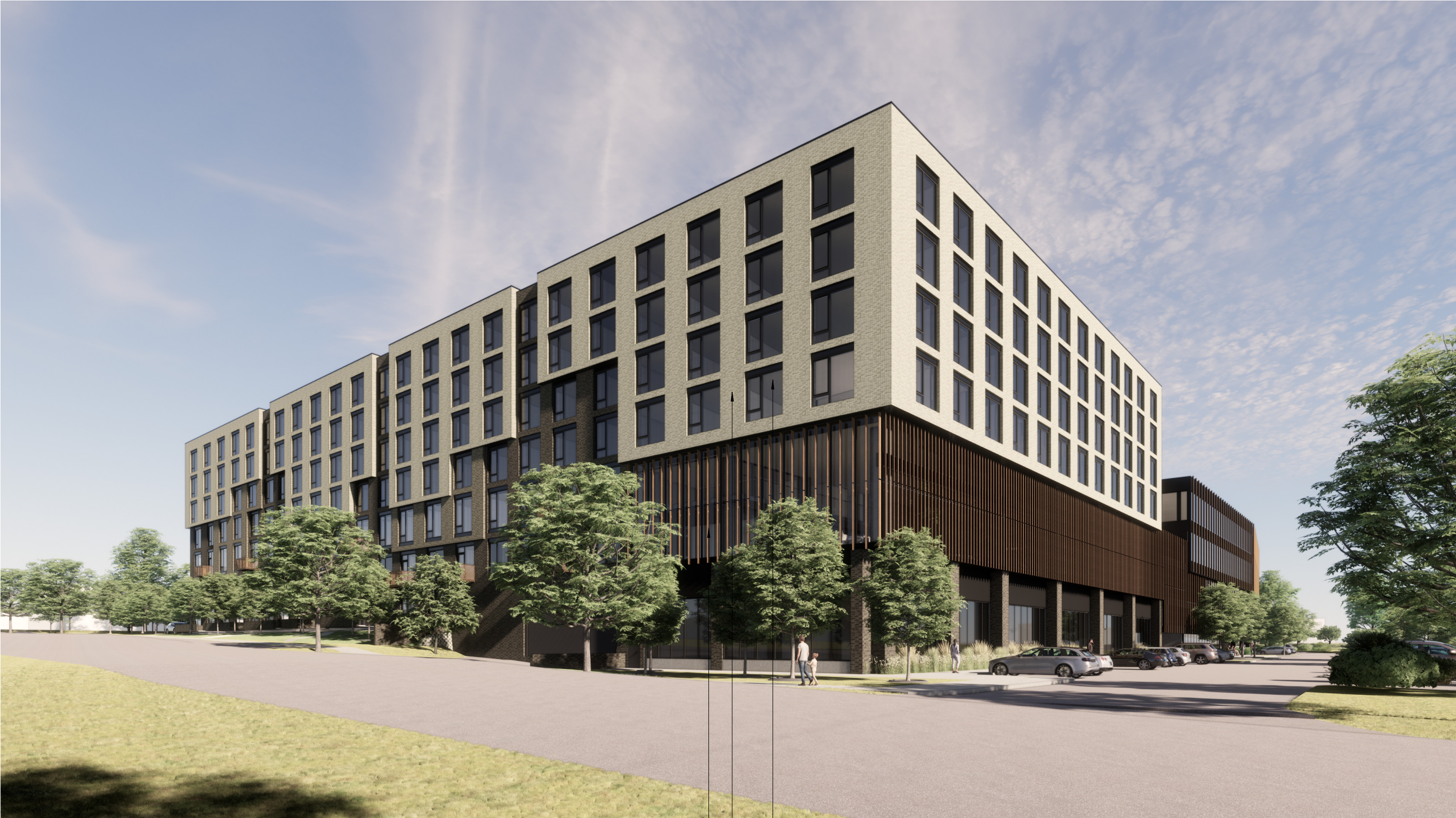
VIEW FROM NORTHWEST ENTRANCE
