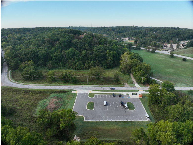
Figure 1: Overall Site View Looking South
