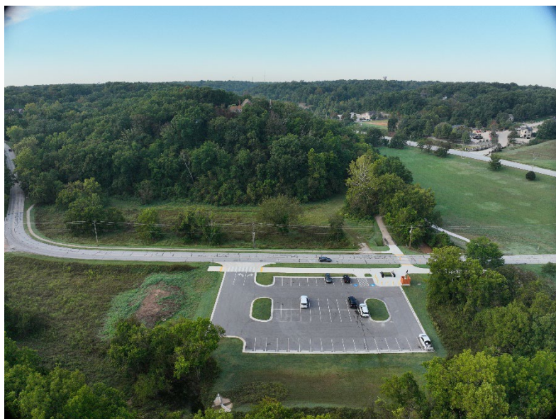
Figure 1: Overall Site View Looking South
