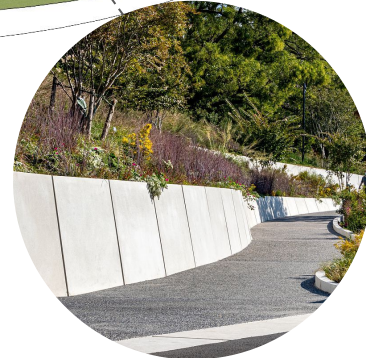
Garden - Path & Retaining Wall
