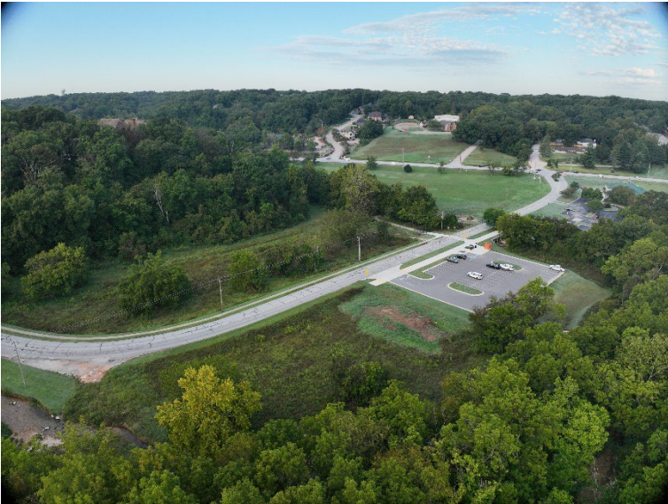
Figure 3: Overall Site View Looking Southwest
