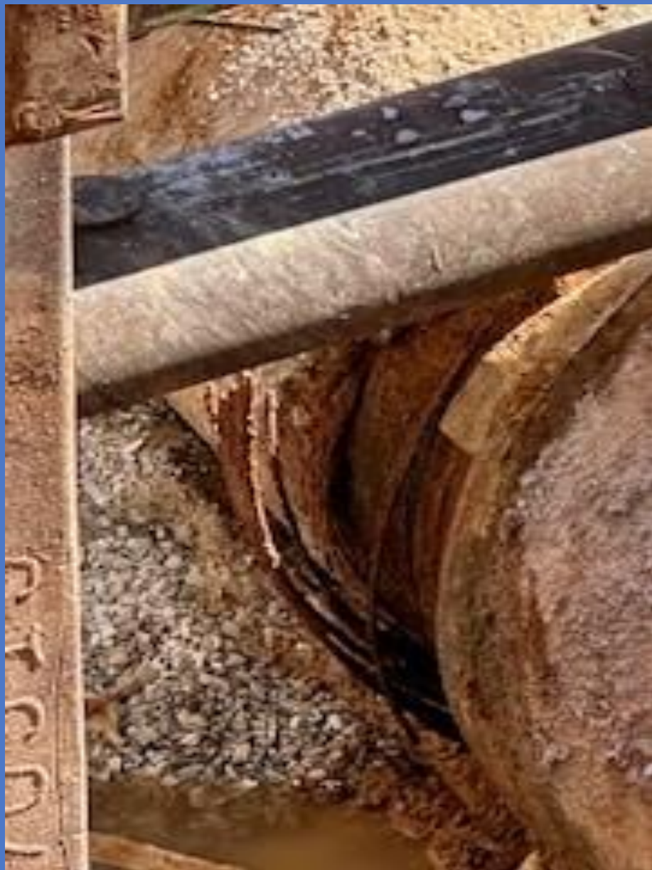
Leaking Joint
