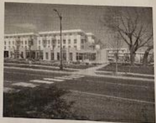
First crossing to the East of the roundabout
