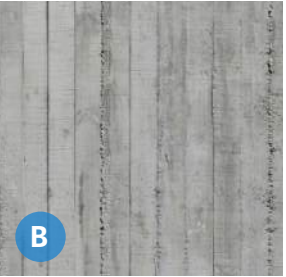
BOARD FORMED CONCRETE
