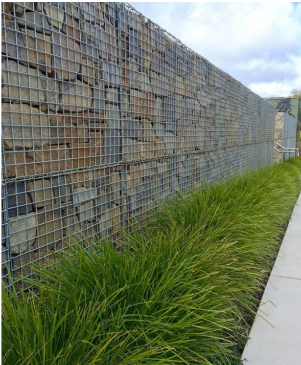
The texture of the stone gives a gabion wall more interest
