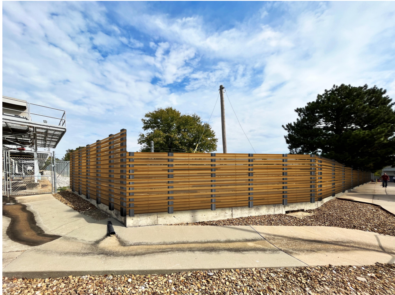
FENCE OPTION TREX FENCE SLATS 4" x 4" x VARIES; GALV. POSTS BOLTED TO THE FACE OF THE EXISTING CONCRETE WALL @ 4'-0" MAX. SPACING
