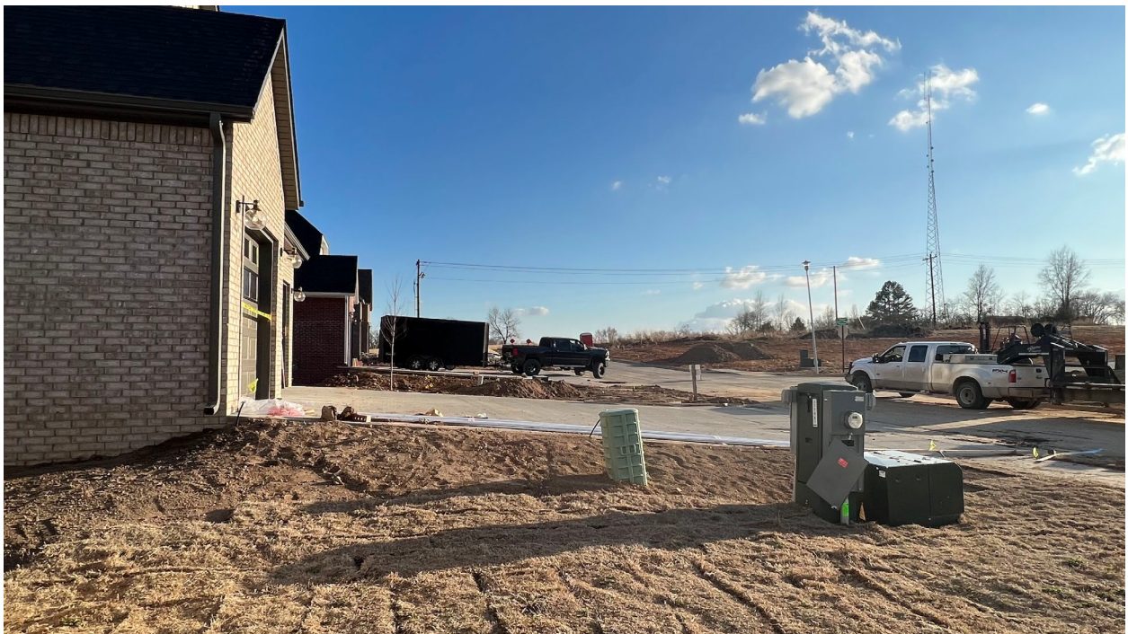
5915 SW Dryden RD house with raised garage height
