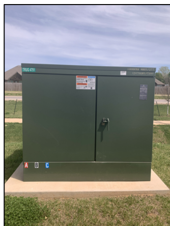
THREE-PHASE PADMOUNT TRANSFORMER
