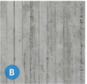
BOARD FORMED CONCRETE
