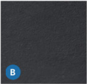
EXISTING PAINTED PRECAST CONCRETE
