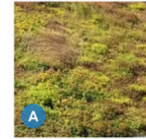
A GREEN ROOF
