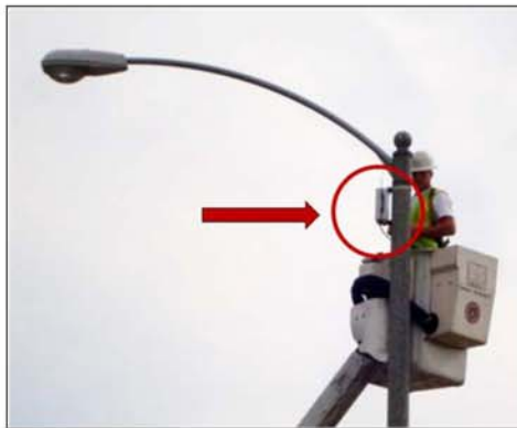
Figure 6 – Typical Mi.Hub collector installation
