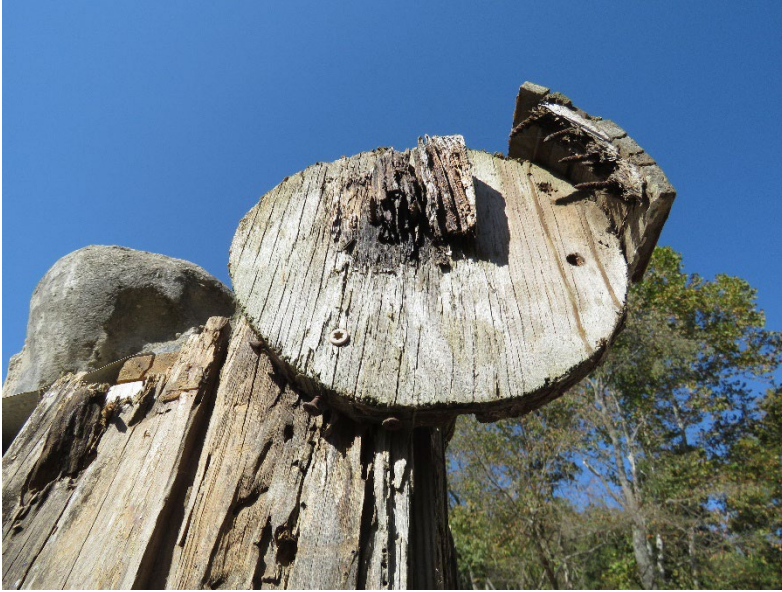
(Left) The deterioration of wood and loss of components have left several screws with their sharp ends exposed. (Right) Some of the deterioration appears to be due to wood boring insects.
