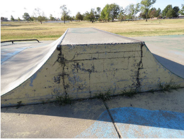
(Left) Cracking on the side walls of a ramp. (Right) The skate park looking southwest, as viewed from the east end.
