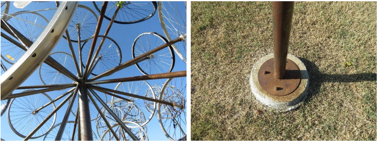
(Left) The pipes of the dandelion all show corrosion. (Right) Corrosion of the stem and self-base, with iron staining on the concrete base.
