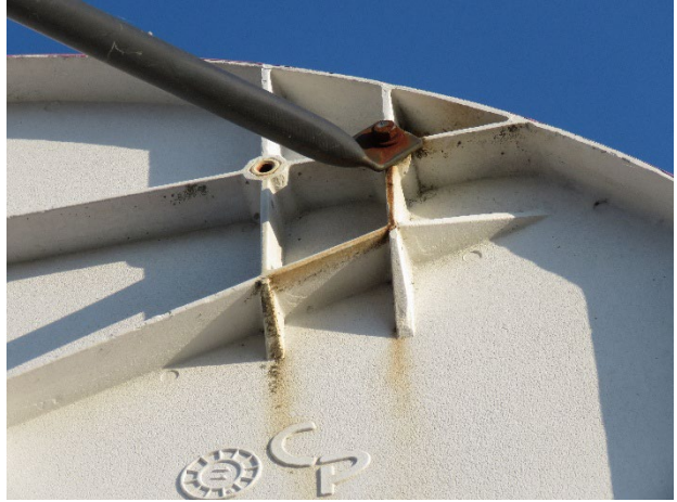
(Left) Cracking and tire marks. (Right) Corrosion of hardware and associated iron staining.
