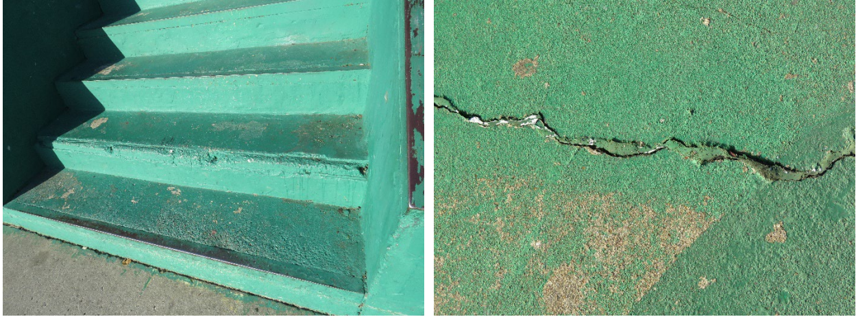
(Left) A missing metal stair nosing. (Right) A crack repaired with sealant, painted to match surrounding surfaces.
