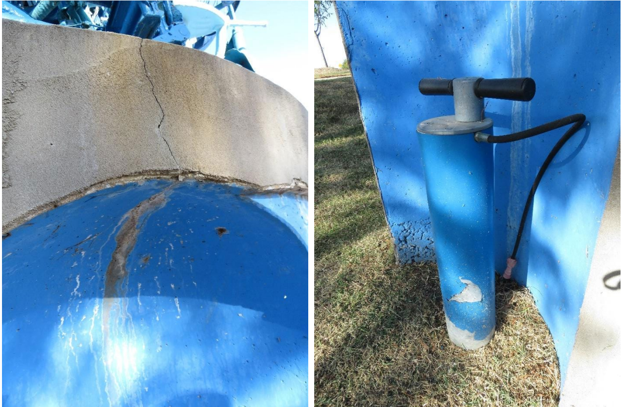
(Left) Cracking in the concrete base, with mineral deposits leaching out of the crack. (Right) Paint loss on the bicycle pump.
