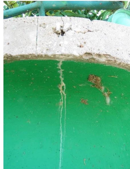
(Left) Pencil graffiti writing on the concrete base. (Right) Cracking around the niche of the base, with mineral deposits.
