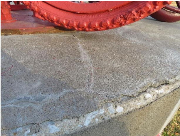
(Left) Cracking in the parging on the concrete base. (Right) Cracking in the painted niche, with mineral deposits leaching out.
