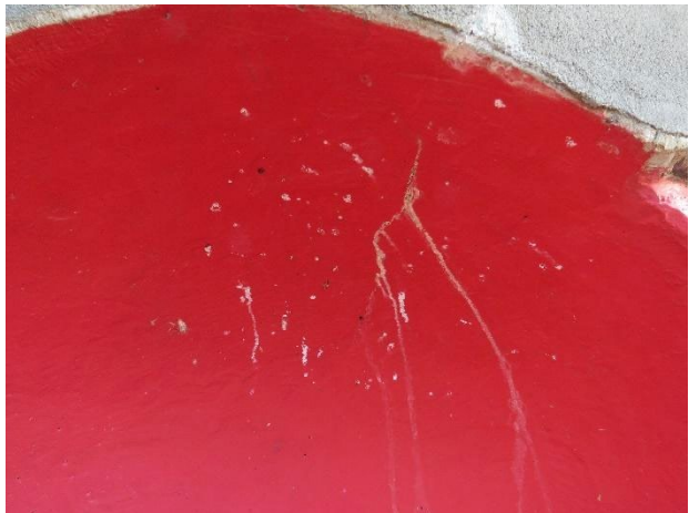
(Left) Cracking in the parging on the concrete base. (Right) Cracking in the painted niche, with mineral deposits leaching out.
