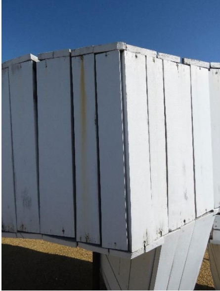
(Left) Displacement of boards and iron staining from corrosion of hardware. (Right) A detached board on the underside, held in place at one end.
