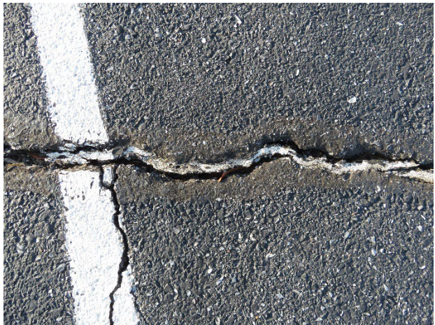
(Left) The 1980s court has large cracks, some of which have been repaired with sealant.
