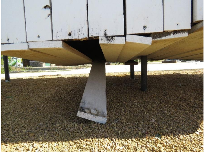
(Left) Displacement of boards and iron staining from corrosion of hardware. (Right) A detached board on the underside, held in place at one end.
