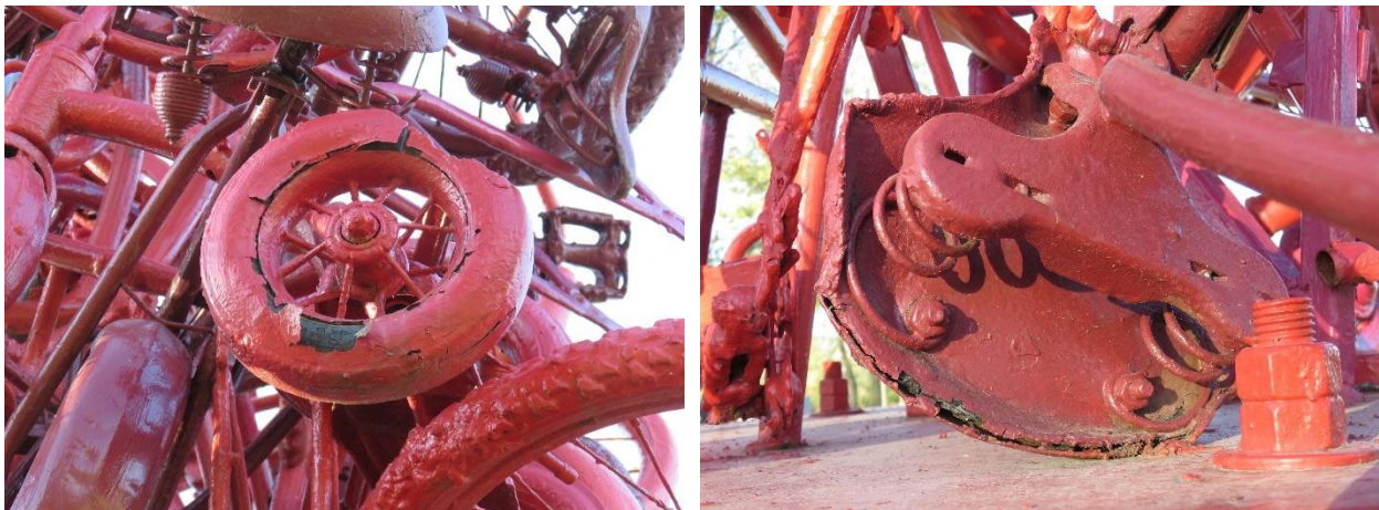
(Left) Losses in the paint coating observed on rubber components. (Right) Breaks/cracking in the paint coating.
