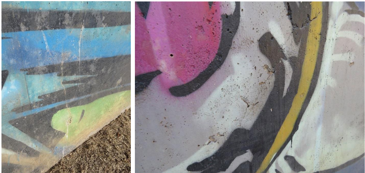
(Left) Cracking in the concrete with mineral deposits leaching out of the cracks. (Right) Voids and cavities in the concrete, small areas where paint did not reach.
