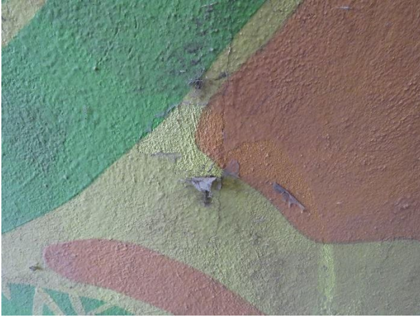
(Left) Actively peeling anti-graffiti coating on the west mural. Note also the heavy soiling on surfaces. (Right) The mural on the east side of the tunnel, identical to the one on the west side.
