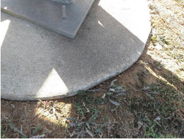
(Left) Numerous chips around the edges of the concrete pad. (Right) Loss of paint on the sign, with corrosion in areas of exposed mild steel.
