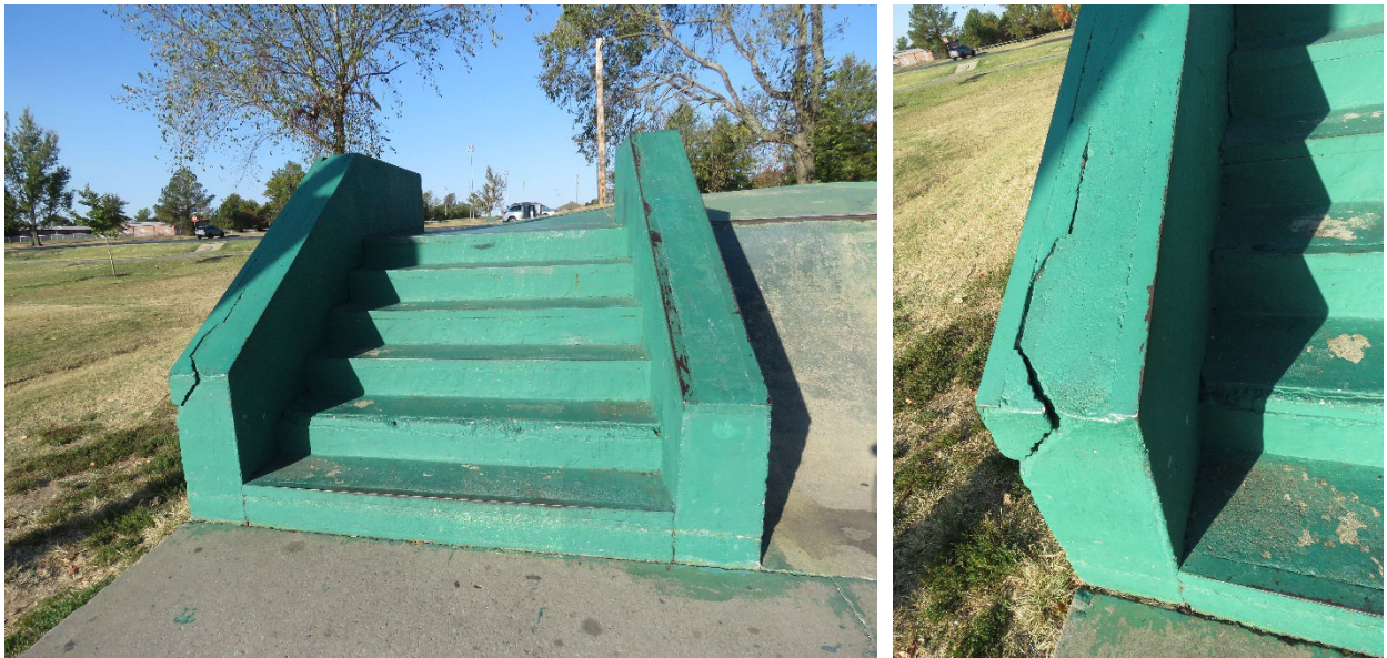
(Left) The stairs located south of the bowl, on the western end of the skate park. (Right) The south concrete bannister exhibits pronounced cracking at top. Note also losses in the paint finishes on the stair treads.
