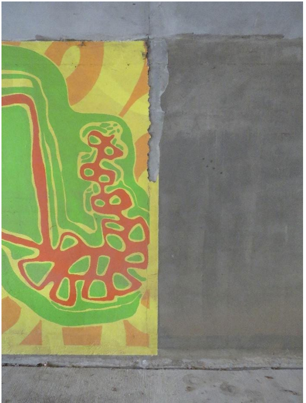
(Left and right) Loss of the parge and paint coats on the side edges of the east mural.
