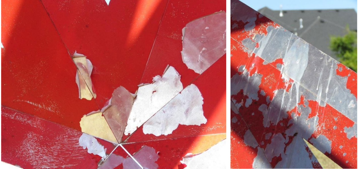
(Left) Actively peeling paint. (Right) Evidence of some type of liquid spilled on the artwork.
