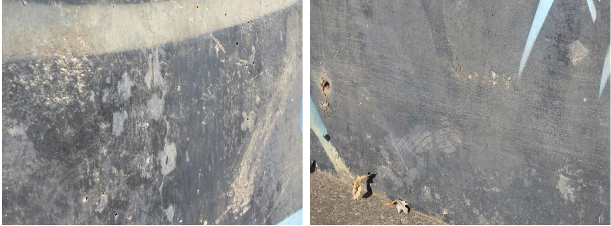
(Left) Cracking in the concrete and bubbling and peeling of the anti-graffiti coating. Note also the heavy soiling. (Right) Linear abrasions on the mural, in an area outside the tunnel.
