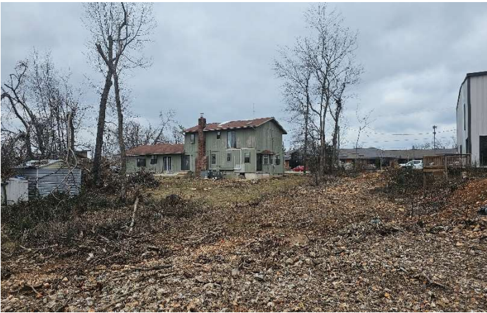
BACK OF 911 FROM EAST NEIGHBORING VACANT LOT
