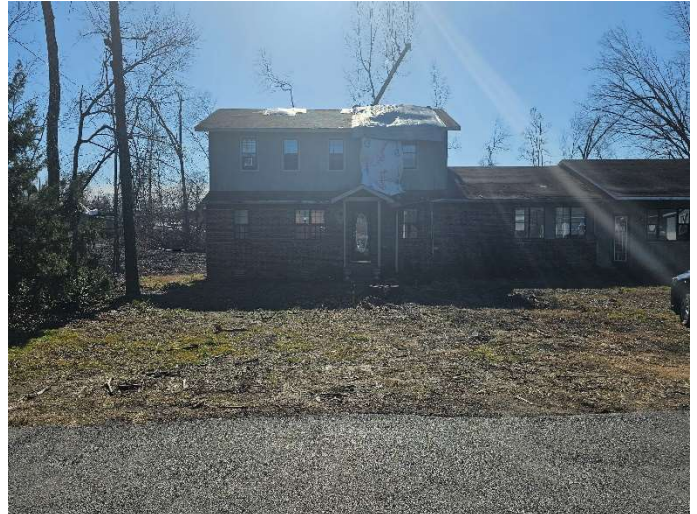
911 FRONT YARD – LOCATION TEMP PARKING
