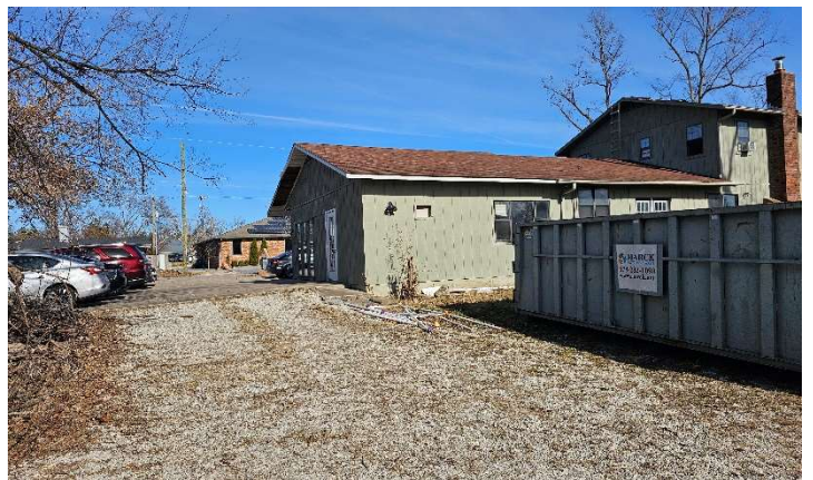
911 NW 7 th BEHIND STRUCTURE LOOKING NORTH TO 7 th
