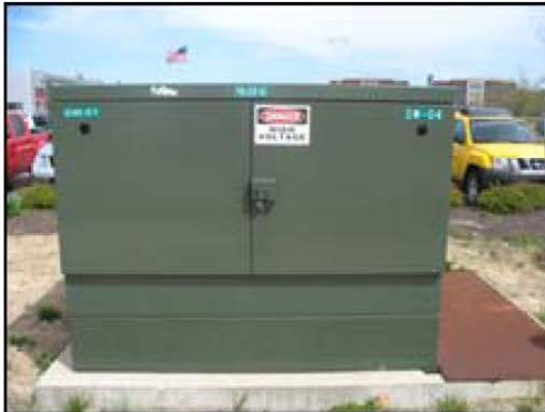
PADMOUNTED SWITCHGEAR
