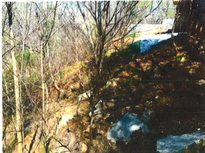
Photograph 1: Looking Along Earth Slope, towards Existing Scarp
