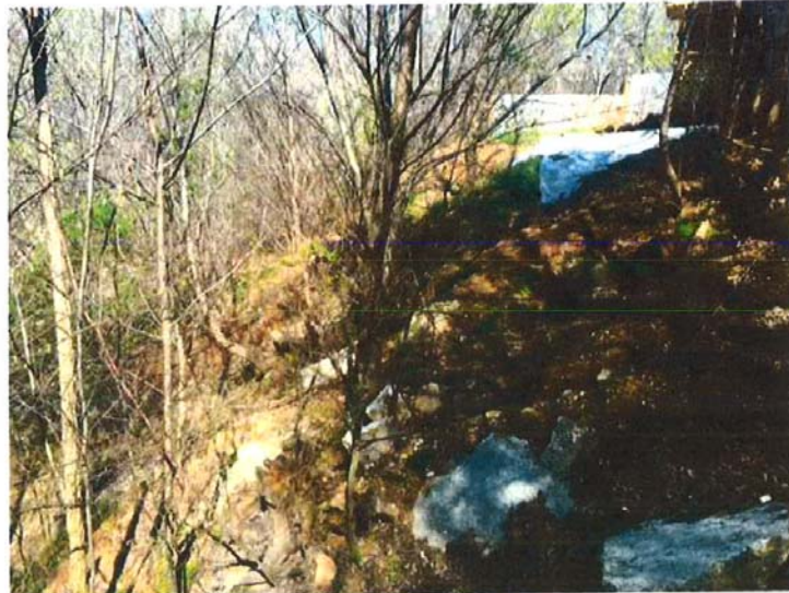
Photograph 1: Looking Along Earth Slope, towards Existing Scarp
