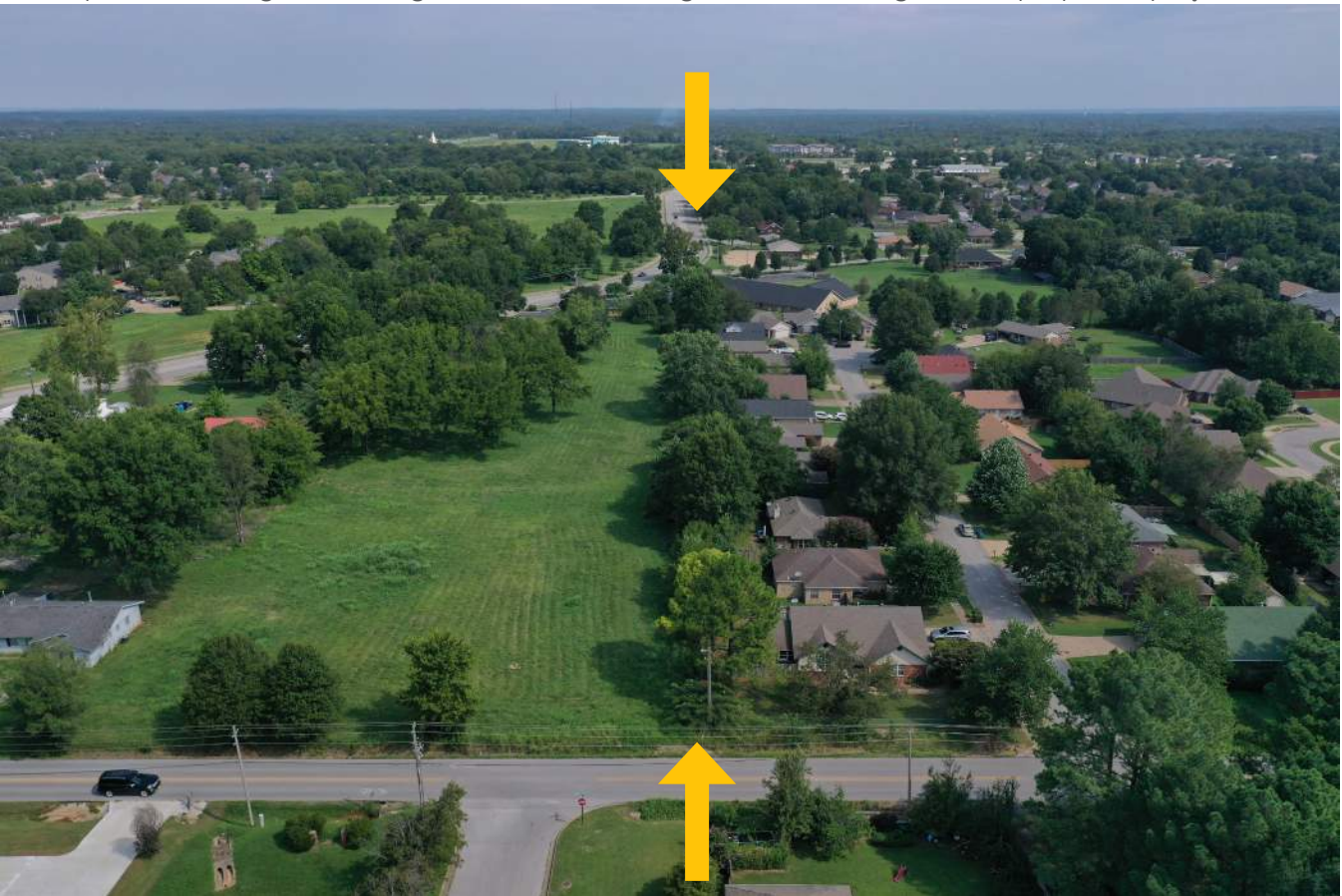
drone photo showing the existing treeline buffer along the eastern edge of the proposed project
