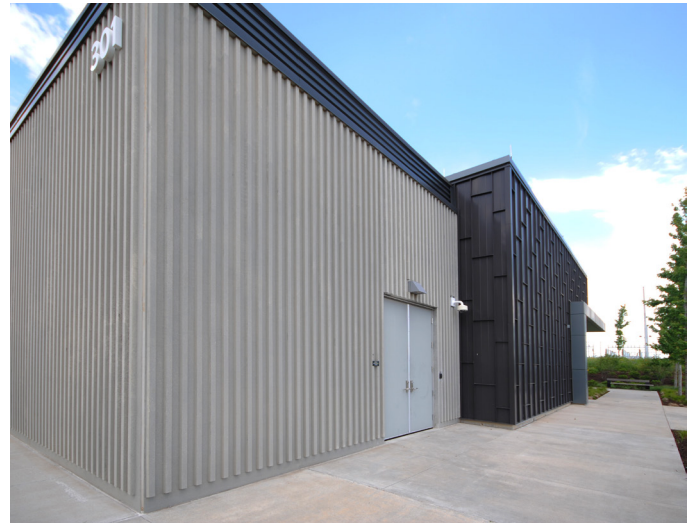
Precast Linear Panel Detail
