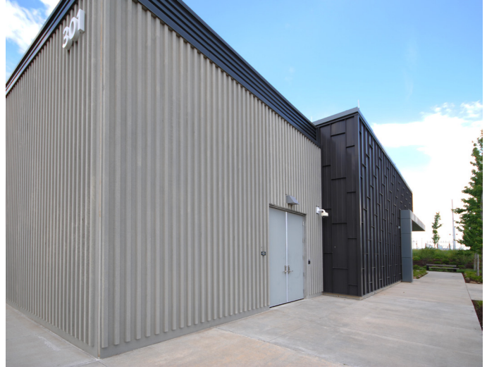
Precast Linear Panel Detail
