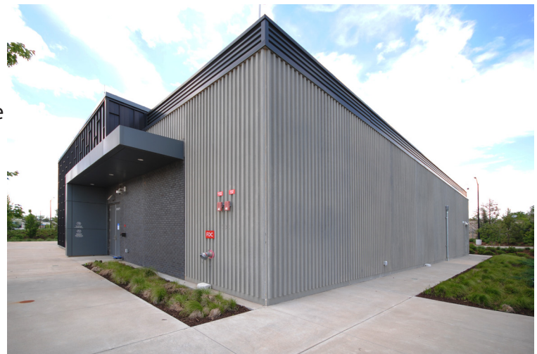
North Central Utility Plant - Precast / Brick Inspiration
