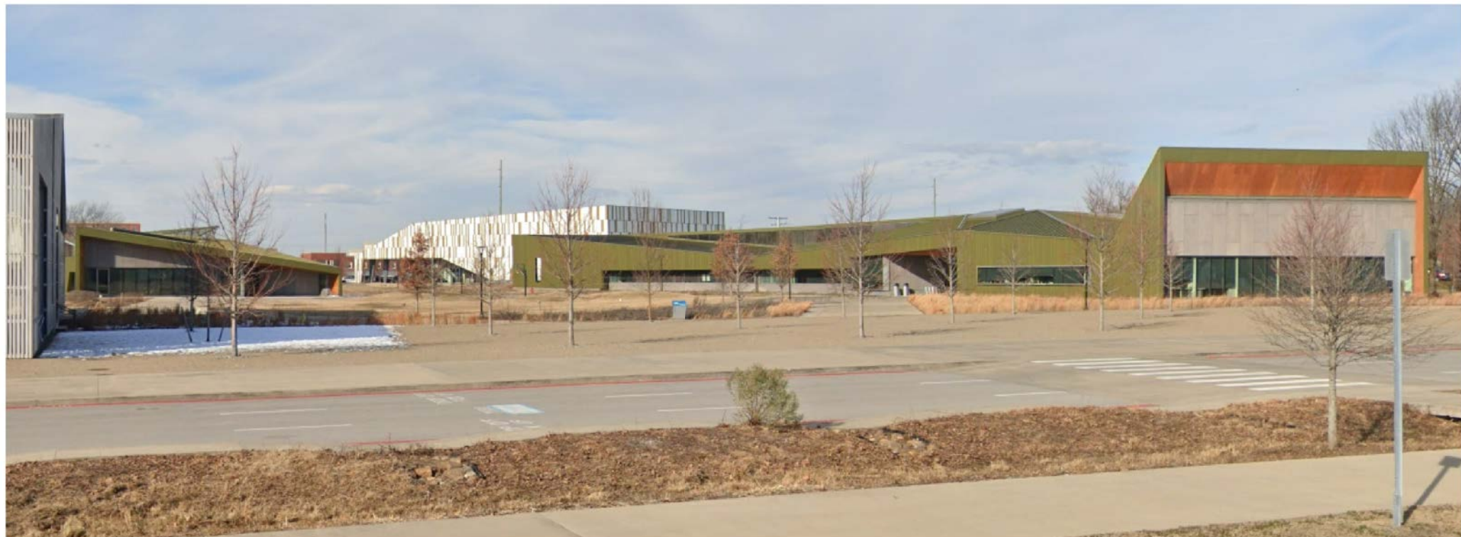
THADEN SCHOOL - 800 SE C STREET
