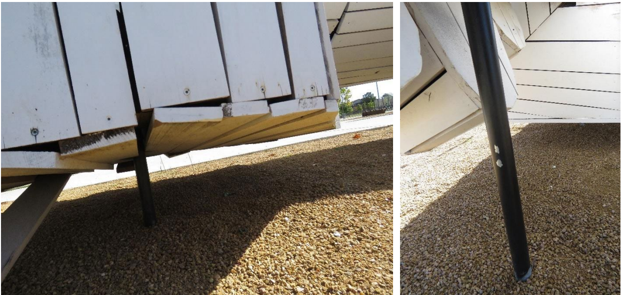
(Left) Warping of boards on the underside. (Right) Localized losses of the paint coating on the metal legs.
