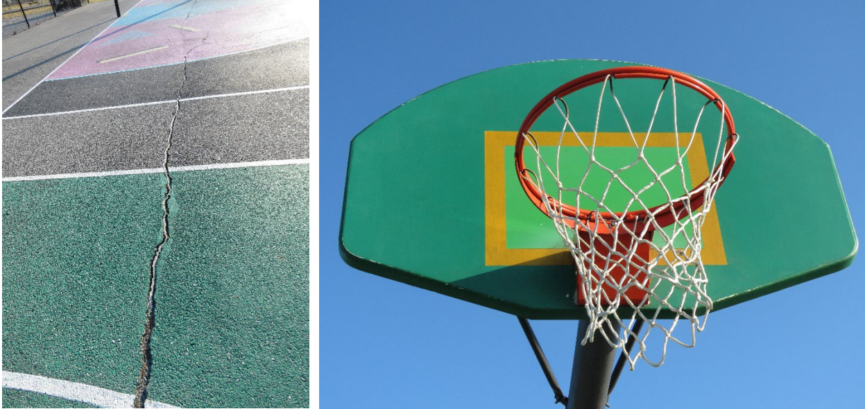
(Left) The crack runs through the 2000s and 1990s court. In some areas the crack is very wide. It has been repaired with sealant, which has failed. (Right) Losses in the paint finish is mostly seen around the edges of the backboard.
