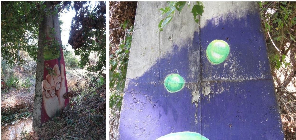
(Left) The third and center pillar is painted on two faces. (Right) Note the peeling and flaking paint on one face, with losses. This is an active condition, and more losses can be expected.
