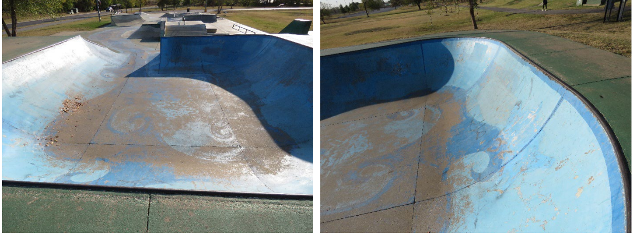
(Left) The bowl, located on the western end of the skate park. (Right) Square patches on the side of the bowl appear to be attempts at covering up graffiti.
