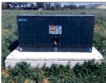
THREE-PHASE PRIMARY JUNCTION BOX
