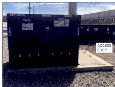
PADMOUNT SWITCHGEAR - MAINTAIN 5' CLEARANCE FROM ACCESS DOOR SIDE OF DEVICE
