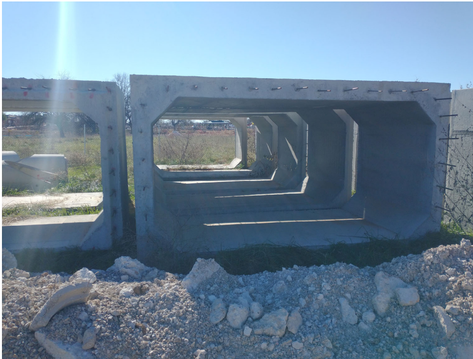
Exhibit Photo: Sample existing box culverts
