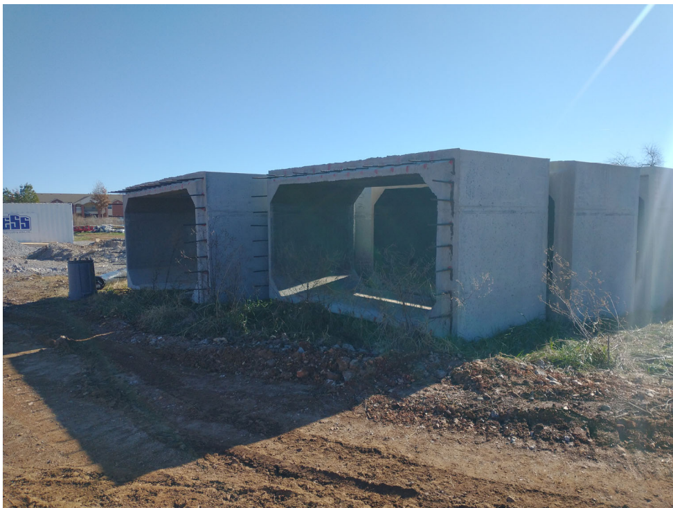
Exhibit Photo: Sample existing box culverts
