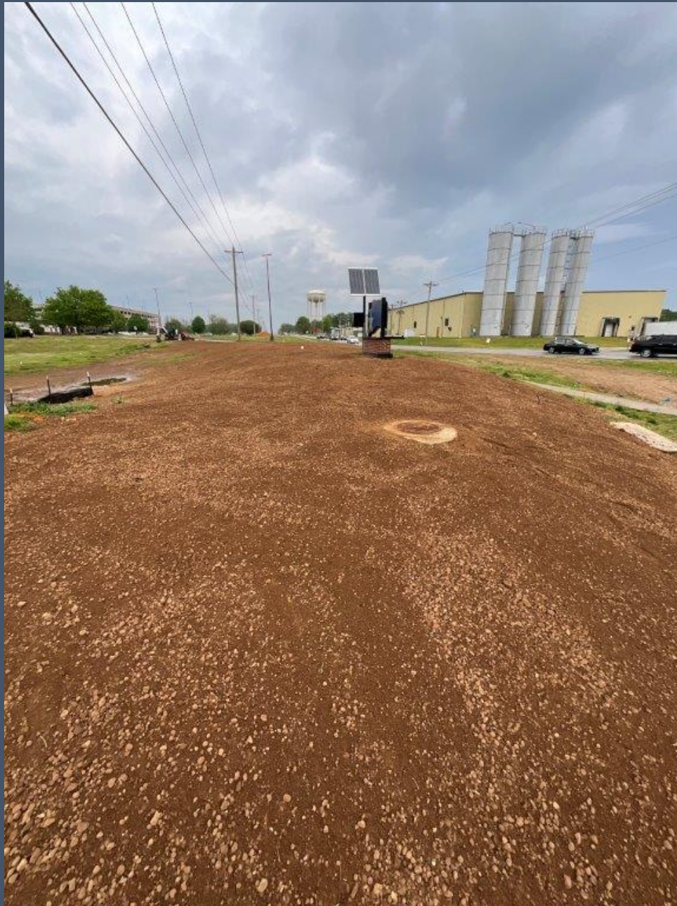
View from southern end of repair site looking north
