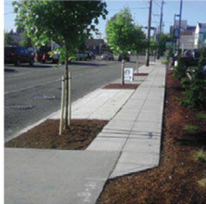
Allows construction of a sidewalk on private property to provide more growing space.
