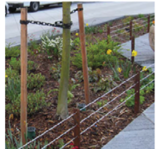
A guard protects the trunk from damage, while rails around the pit help prevent soil compaction.
