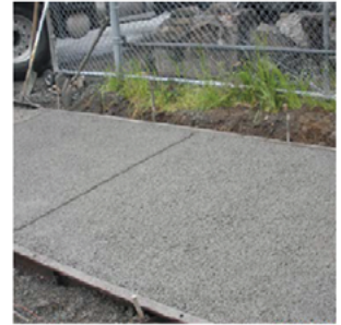
By allowing air and water to pass through to the soil below it may deter shallow root growth.
