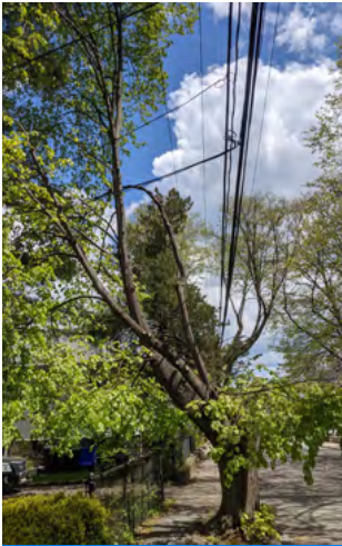
Overhead Utility Conflicts
