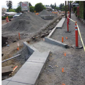
An open-graded gravel base course under the sidewalk to discourage root growth.
