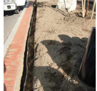
A barrier, often plastic, that deters root growth near the surface.
