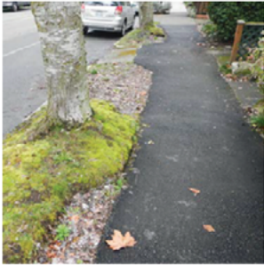
A cheaper, flexible sidewalk fix, but requires more upkeep and doesn't last as long as concrete.
