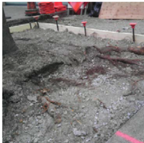
Removal of roots damaging sidewalk damage, overseen by a qualified arborist.
