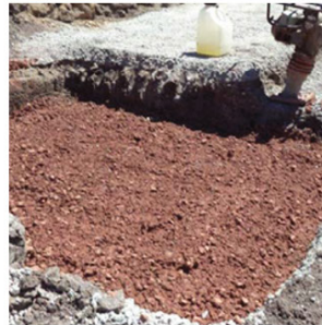
Specially designed to provide space and porosity while still supporting pavement
