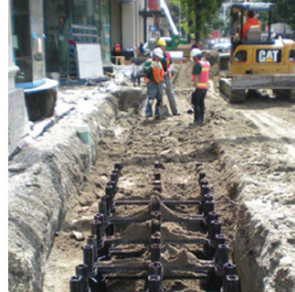
Structurally supported pavement that still provides space for roots to grow.
