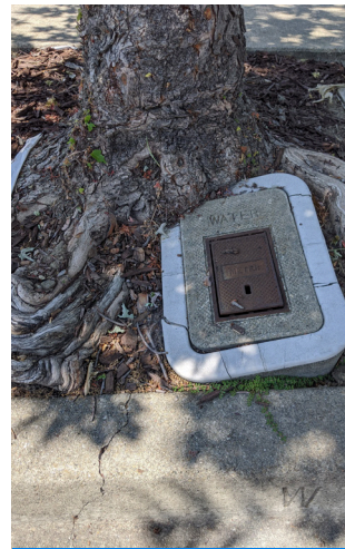
Underground Utility Conflicts
