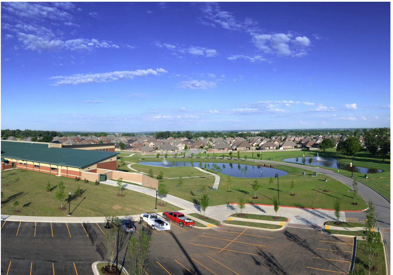
Existing parking lot of MPL-3 (Source: Halff)
