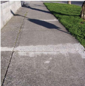
Cutting down raised concrete edges to reduce tripping hazards.
