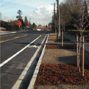
A shift in curb location for that widens the planting strip, often for whole blocks.
