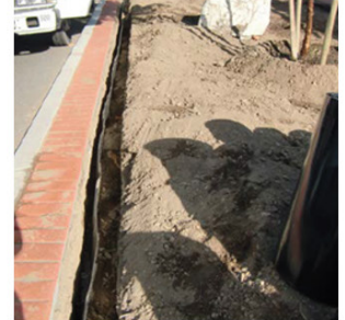
A barrier, often plastic, that deters root growth near the surface.
