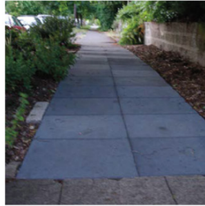
A flexible surface that offers room for continued tree root growth under the sidewalk.
