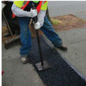
A temporary measure to smooth a cracked or lifted sidewalk, typically done with asphalt.
