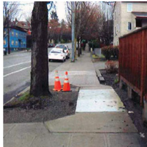
A section of sidewalk that supports itself from the ends, on piers, without the need for compacted subgrade below.
