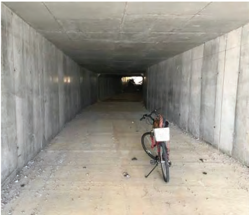
1) On the north side of the tunnel along the Razorback Greenway, there is ample space between the bridge and the area known as Blue Hole to accommodate a public art installation. Note: A stream restoration project is planned for 2027 in this area. Any proposed artwork should be located and designed with the planned restoration in mind to avoid future conflicts.
